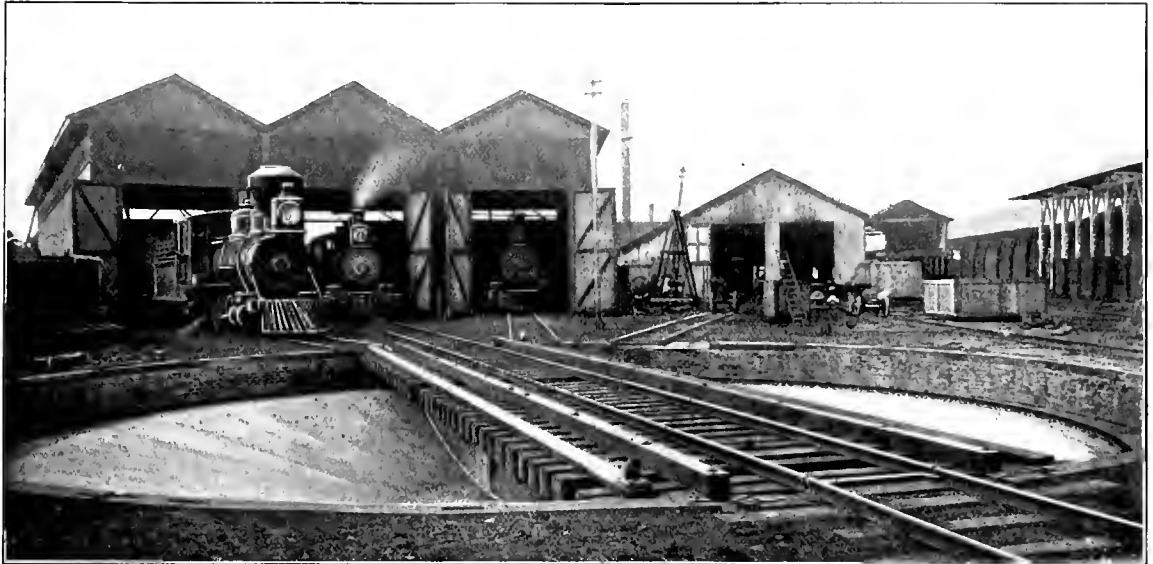
ENGINE HOUSE AND REPAIR SHOP, SANTA ANA RAILROAD.
